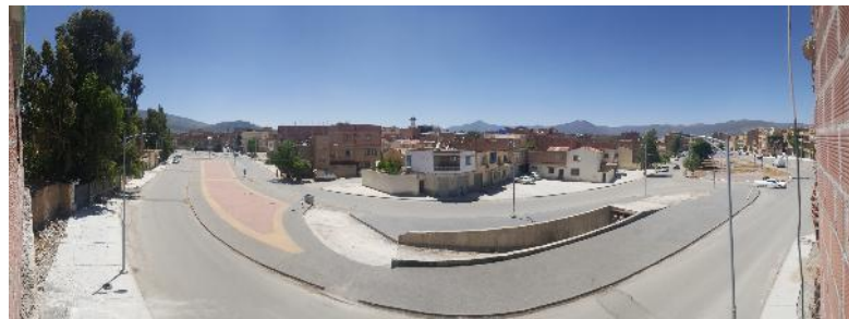
Fig. 3– A panoramic view of the entrance to the informal settlement after the completion of the development works
