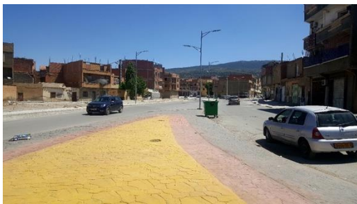
Fig. 4– A photo taken of part of the neighborhood showing: street lighting, easements for household waste and a highway. Houses for sale and others under construction.
