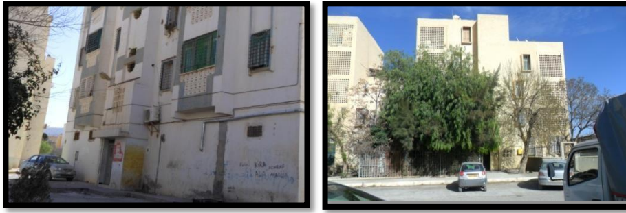
Figure 4.91. Parking in front of the building entrances.
