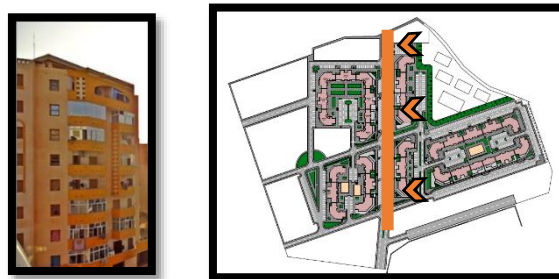
Figure 4.130. The closing of the balconies.
