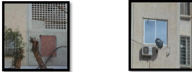
Figure 4.95. Closure of balconies and dryers and change of window joinery
