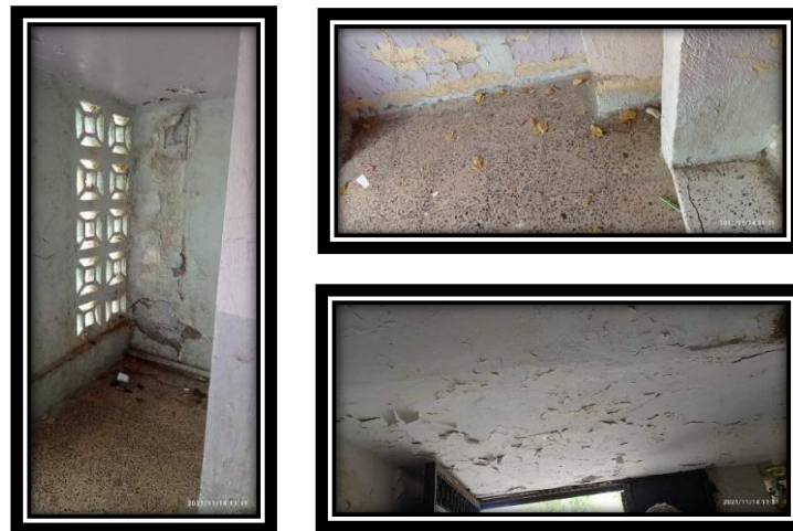
Figure 4.101. the entrance hall.
