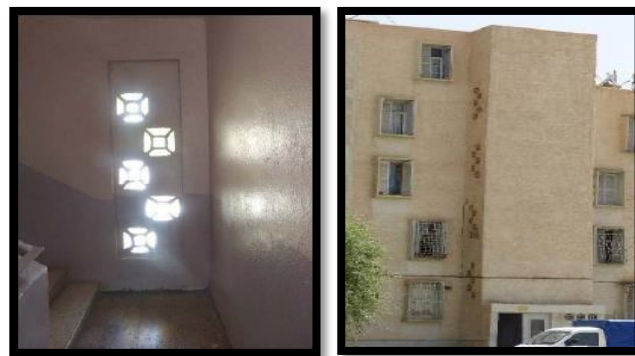
Figure 4.99. The stairwell seen from outside and inside.
