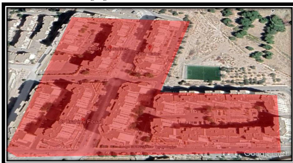
Figure 3. 14. The 1000 housing units AADL in Bouzourane Batna.
